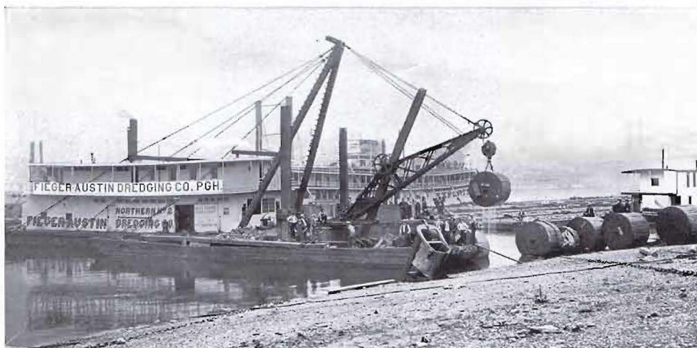
Floating dredge, rigged with 1-inch Yellow Strand Powersteel Wire Rope, loading twelve submarine cables for high tension system under Ohio River at Pittsburgh.
